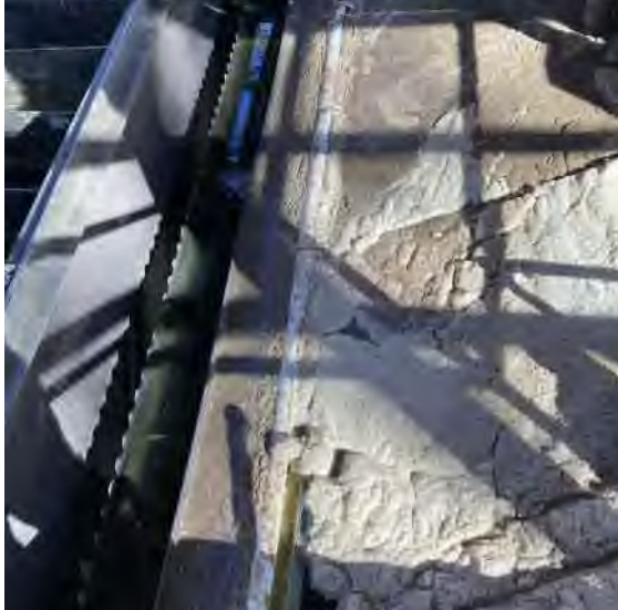
Scum collection pipe and clarifier weir
