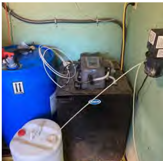
Sodium Hypochlorite (12.5%) feed and composite sampler.
