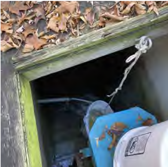
Dechlor tablet feeder, sample collection point, and cascade steps.
