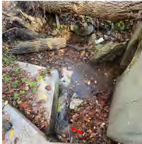
Red arrow is pointing to Outfall 001. The photo also shows a storm drainage outlet and blockage in the stream caused by fallen trees.
