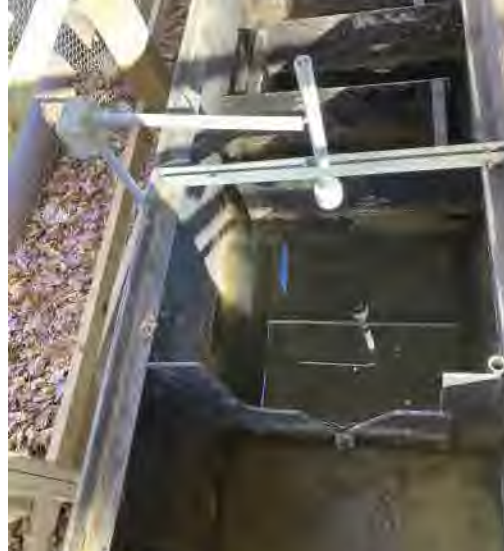
Chlorine contact tank, ultrasonic transponder, and weir.
