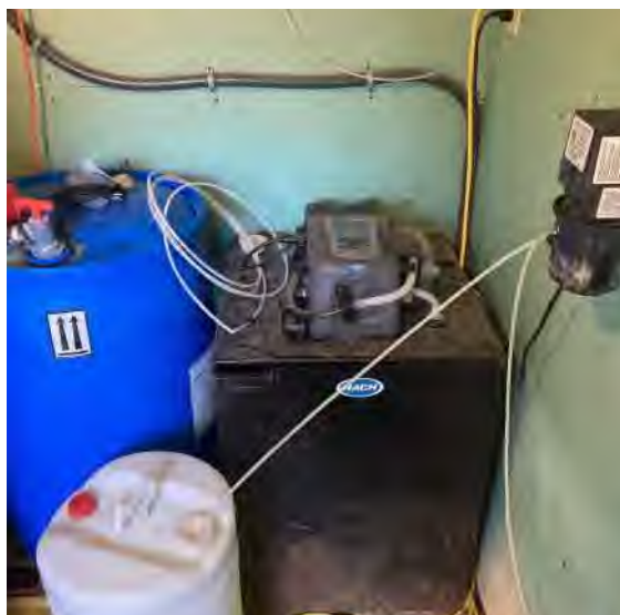
Sodium Hypochlorite (12.5%) feed and composite sampler.
