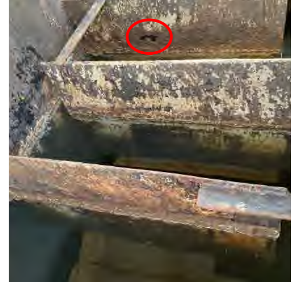
Baffles of chlorine contact tank. Circled in red is a hole developing from rust.
